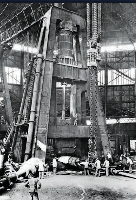
Photo 1: 108-tonne big power hammer - 1909 (period photo)
